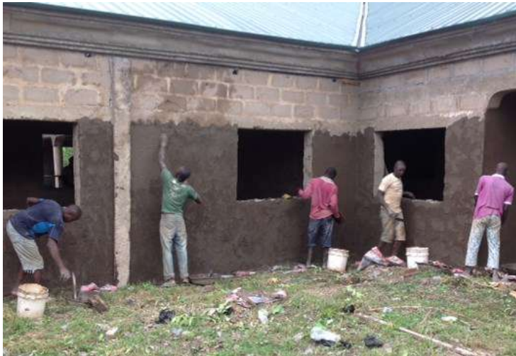
The Medical Centre, Lokoja. Plastering work is nearly finished!
