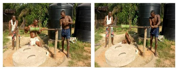
The holding tanks for well water have to be cleaned out at the same time. Notice the piles of silt.
