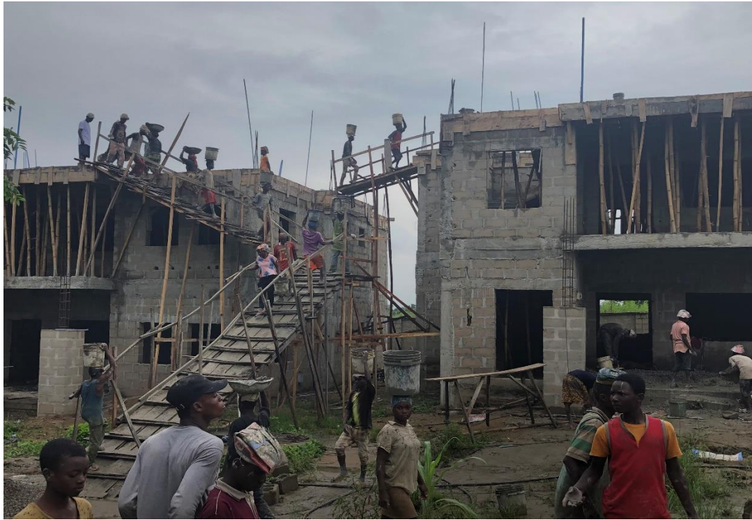
Decking of the 2nd suspended floor of the two residential buildings in progress
