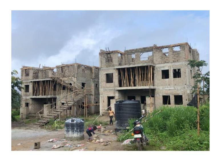
Also, we have made significant progress in our kitchen/dining building which has been redesigned to accommodate two more floors to be used as classrooms. We finished iron and concrete work for the first suspended floor and will commence walling soon.
