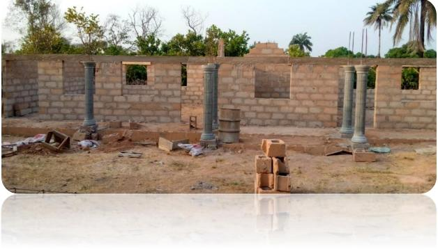
Work on the laid down foundation of four classroom block has begun, the Mason, iron bender and Piller molder came and worked this January and the structure has been built to the lintel level.
